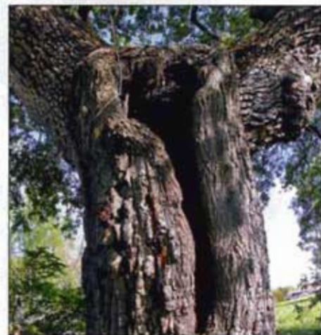
Avoid retaining trees with significant structural defects where damage or injury would occur if they failed. The extensive trunk cavity at the junction of the scaffold branches is a defect that makes this tree unsuitable for preservation.
